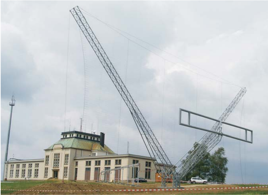
AHR 1/1/0.2 Rigid Dipole Antenna (Picture by courtesy of RTL Luxembourg)
