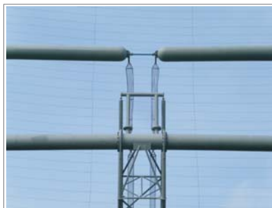
Dipole feed point
